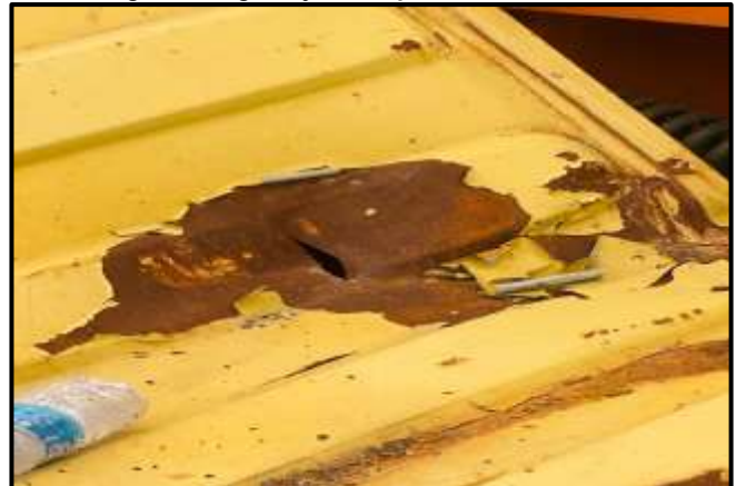
View of the roof panel of container found perforated
